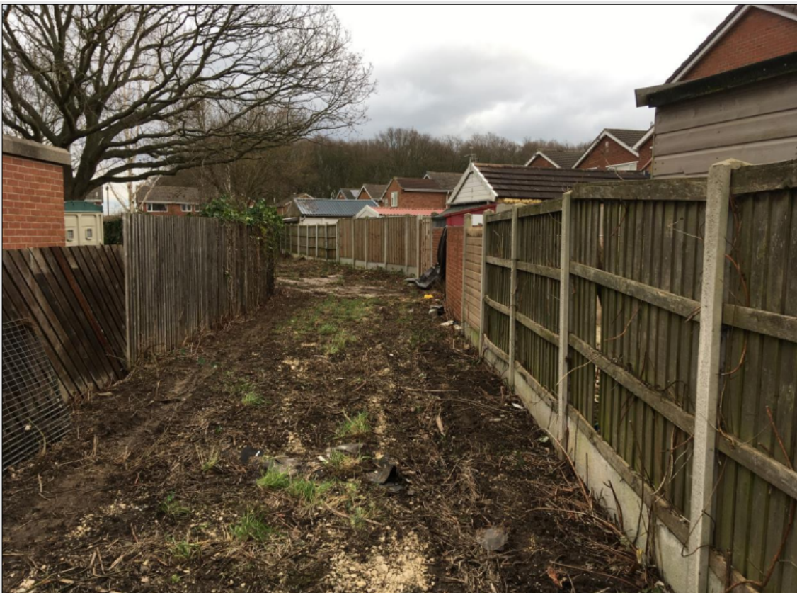
Photo 2: Application Site - access track
